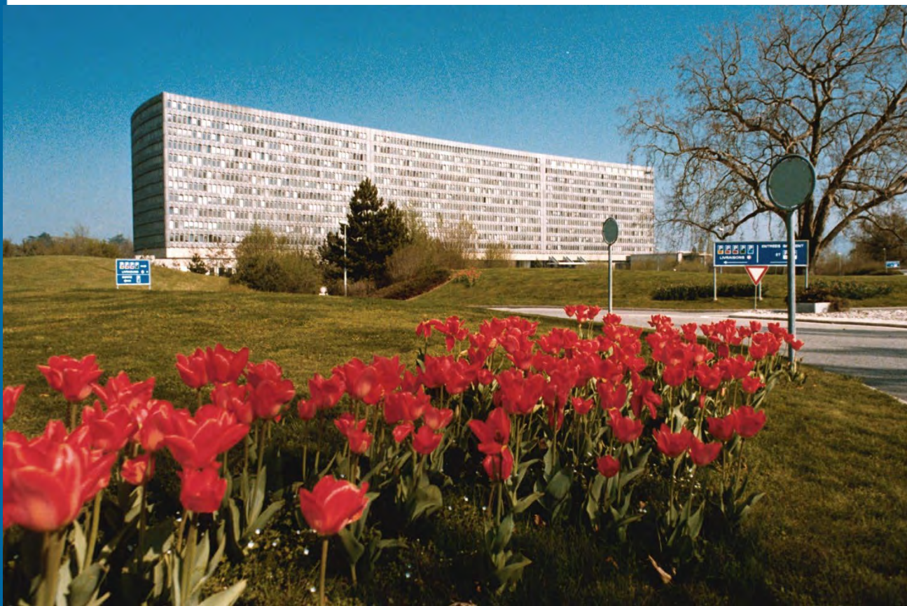
ILO building in Geneva
